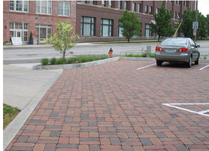
Pervious parking lot
