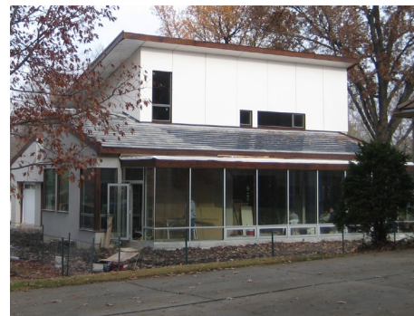
Solarium and windows strategically located at south elevation with overhangs
