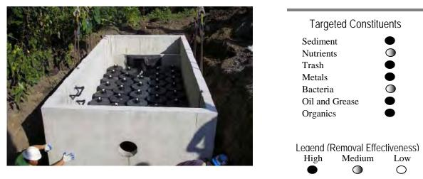
Picture Source: CONTECH Stormwater Solutions Inc.
